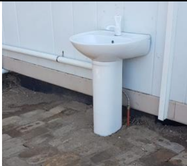
New external basin installed for hand washing
